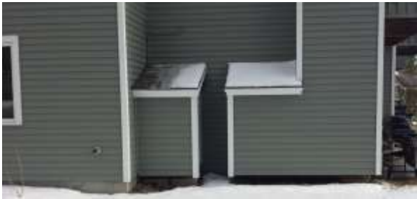
Units 19 and 20 – Kerosene (Side)
